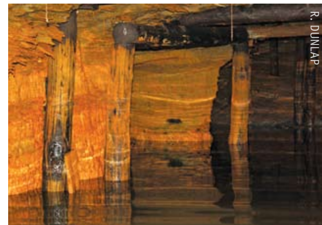
Deep mine in the Kettle Creek watershed, Clinton County
