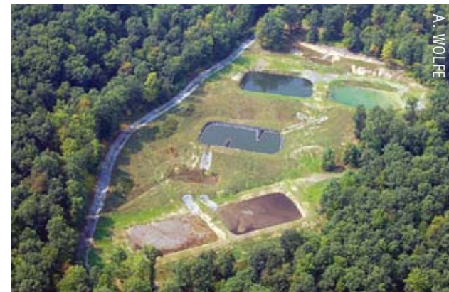
Middle Branch passive treatment system
